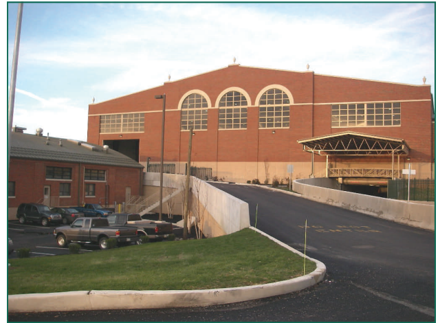
Transfer Building in Manheim Township, Lancaster County, PA
