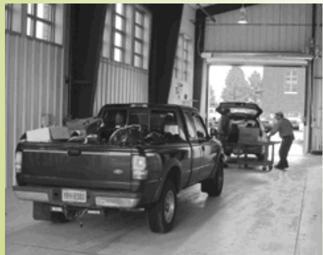
Drive-thru Household Hazardous Waste Facility
