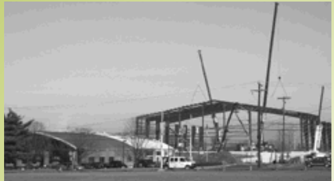
Shell of the new Transfer Station building beside the office
