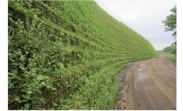
Example of MSE Berm at Lanchester Landfill
