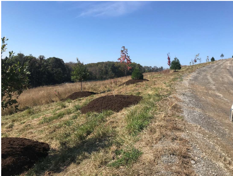
Photo 6 – Crown Excavating completed mulching around planted trees.
